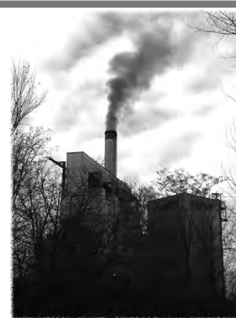
Photo of visible emissions from the LWEC smoke stack in November 2015, just two months after a failed stack test.
