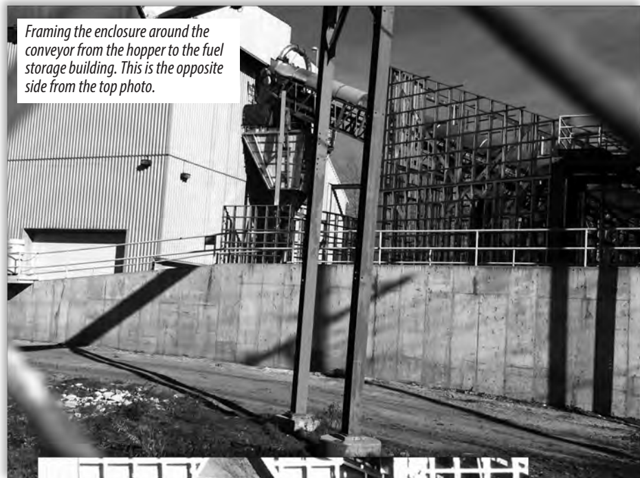
Framing the conveyor partial enclosure, which is supposed to reduce toxic fugitive dust.
