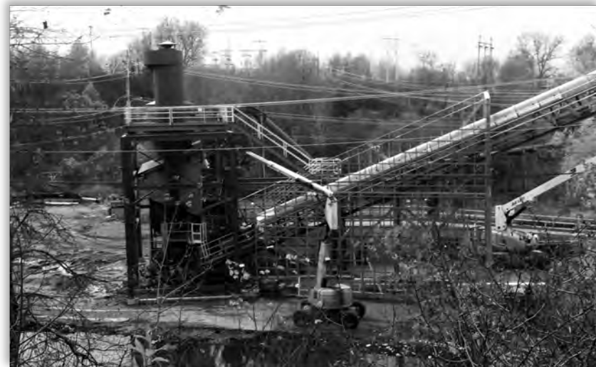
Framing the conveyor partial enclosure, which is supposed to reduce toxic fugitive dust.
