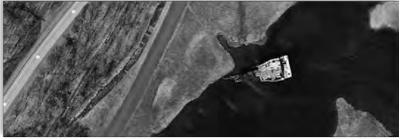
Satellite image of the dredge, sitting in the south end of Torch Lake.
